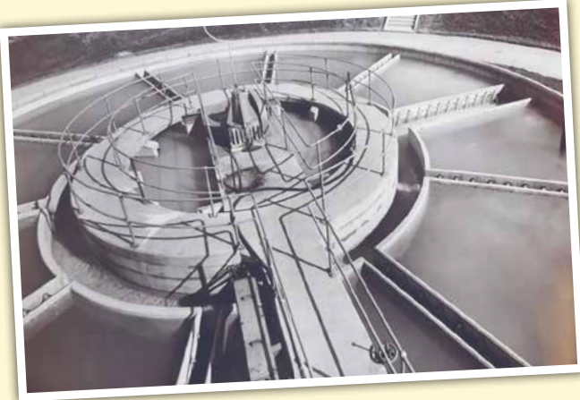
While amalgamating with other companies, Bristol Waterworks continued to innovate in water treatment. The Accelerator introduced at Stowey in 1954 was a state-of-the-art clarification and water softening plan.
